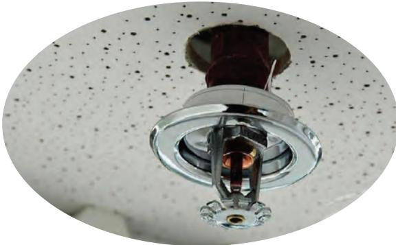
*It is a fire fighting system for protecting structures against Fire. Purpose of using Sprinkler System is to eliminate Fire Condition by flowing pressured water before it develops. Sprinkler Head is placed in wall or ceiling, other end of sprinkler is connected to pipes. It is triggered when the heat exceeds temperature limit of heat sensor bulb in Sprinkler Head.*
